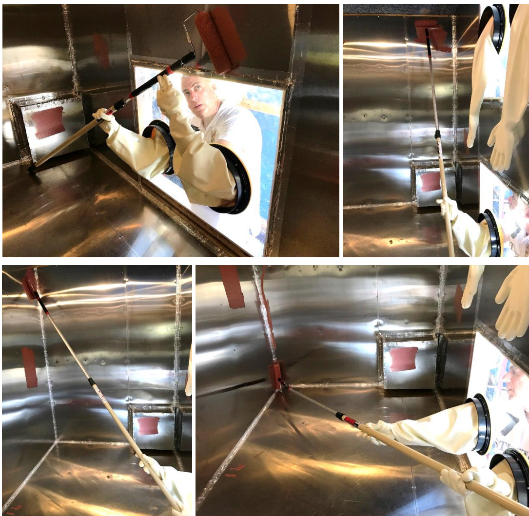
Figure 17. Testing ability of reaching all hot cell surfaces from lower glove ports using a manual long-reach tool outfitted with a roller for applying intumescent coatings.
