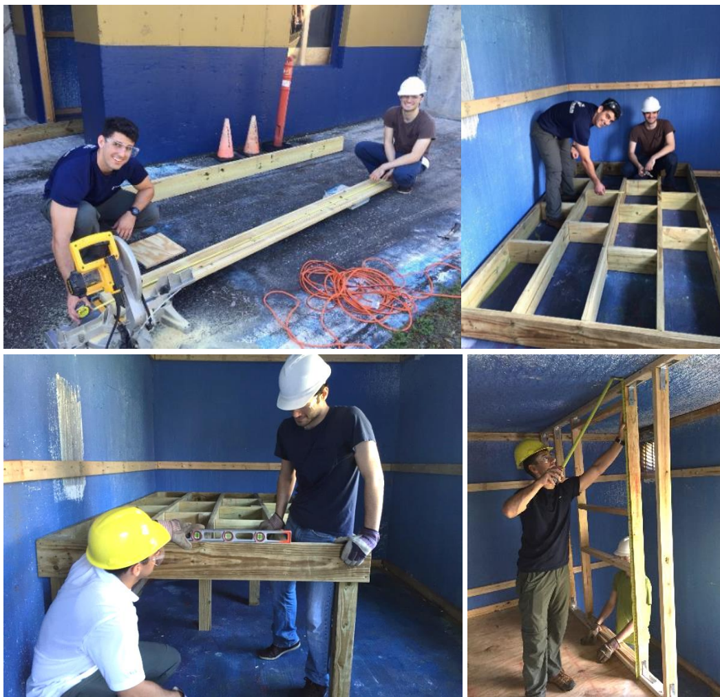
Figure 14. Construction began on the selected hot cell mockup design.
