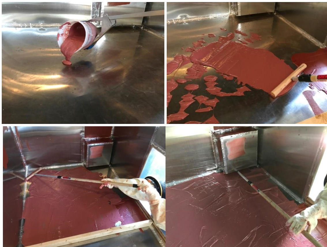
Figure 20. Slow pour method to apply IC to hot cell floor.
