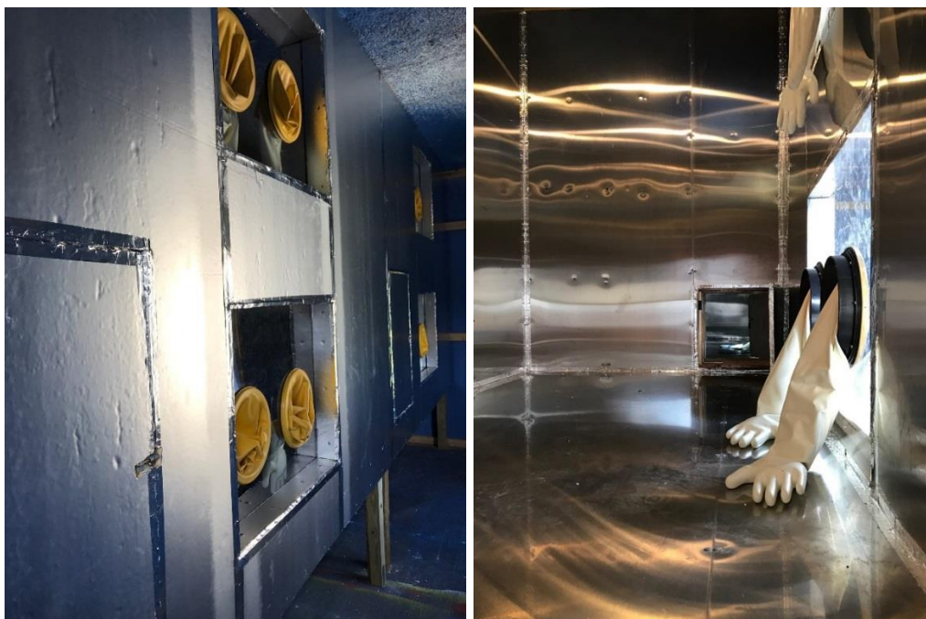
Figure 15. Completed construction of Hot Cell Test Bed at ARC.
