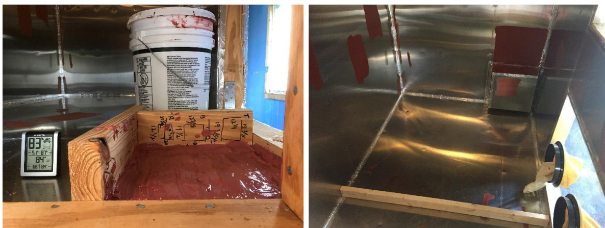
Figure 18. Small scale test of a slow pour technique using intumescent coatings (left) and preparing for full-scale demo of slow pour application method for horizontal / floor surfaces in hot cell (right).
