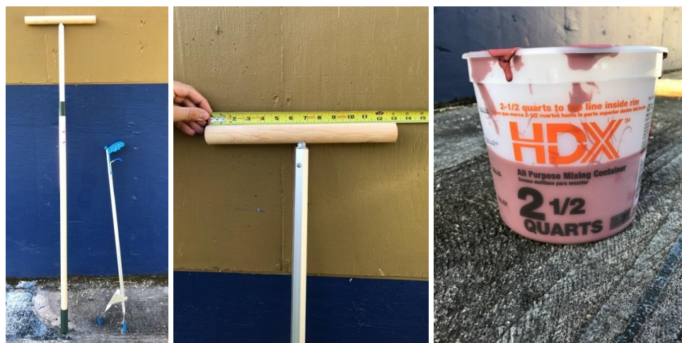
Figure 19. Tools used for slow pour method to apply IC to hot cell floor.
